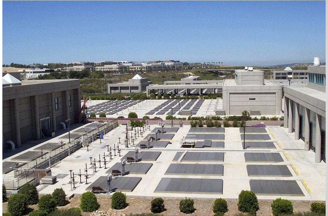
North City Reclamation Plant located in Mira Mesa. Source: City of San Diego Public Utilities
