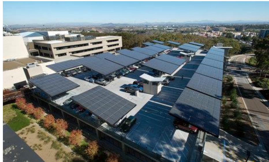
Photovoltaic “grove” on the roof of Hopkins garage. Source: University of California, San Diego
